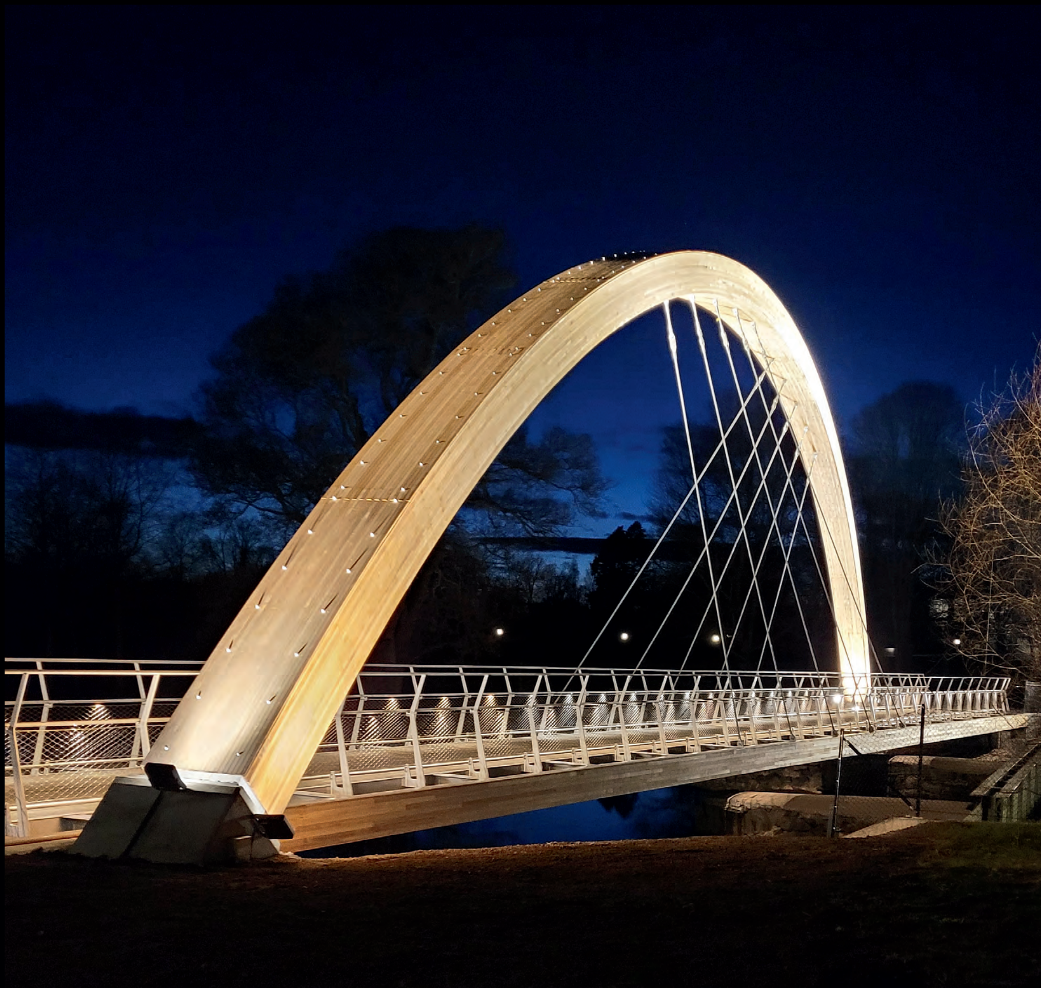
Sweden – Björkbornsbron Bridge, Karlskoga
